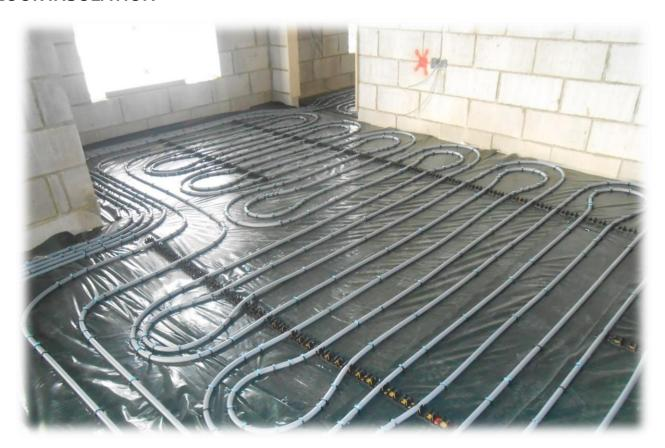
Thermal Surfaces underfloor heating/cooling systems can be incorporated in to any type of floor construction that has a floor screed above it.
