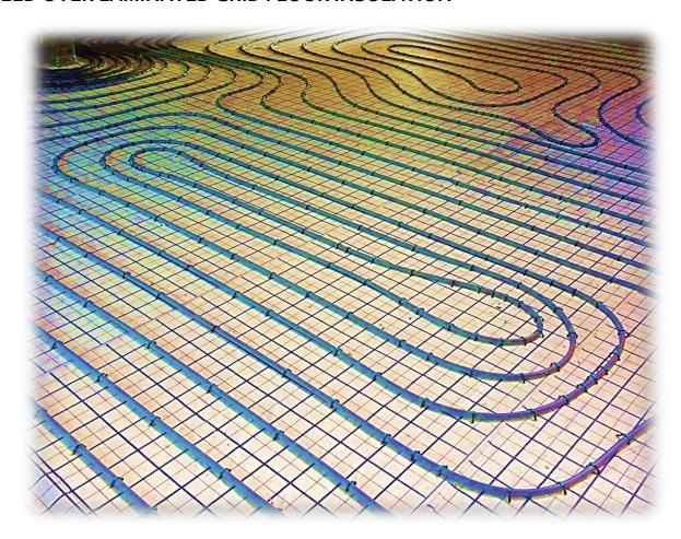
Thermal Surfaces underfloor heating/cooling systems can be incorporated in to any type of floor construction that has a floor screed above it.
